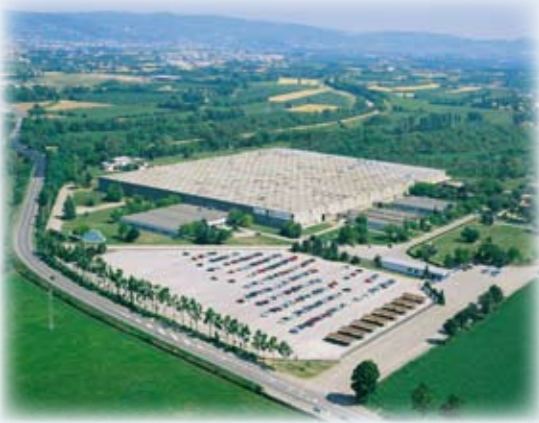
Manufacturing Plant Arzignano - Italy
