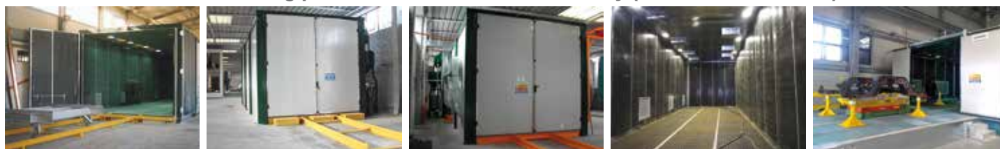
With base and track inside the building
