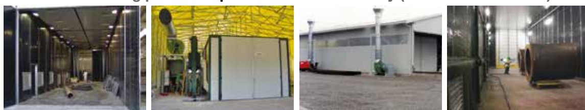
With loading hopper inside the building
