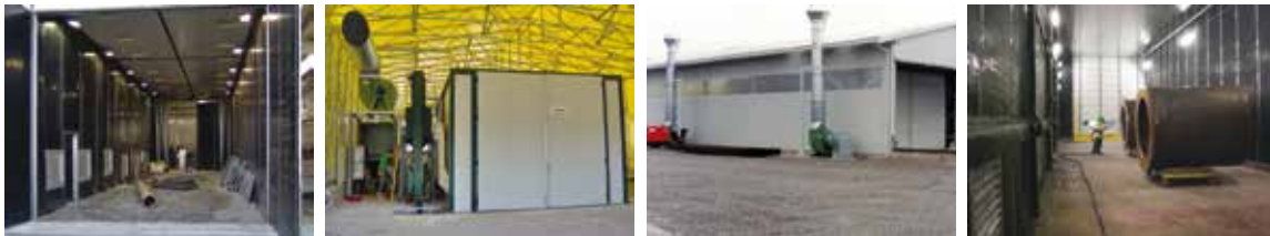
With loading hopper inside the building
